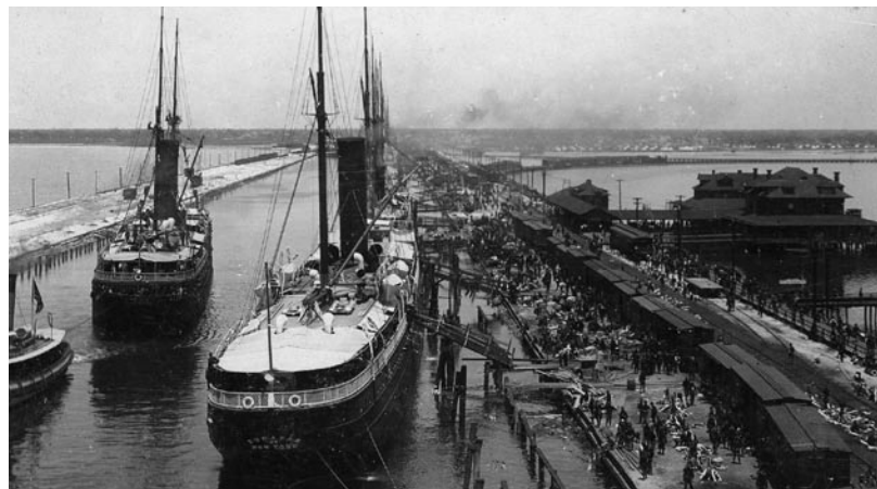
Ensminger photograph taken in Stanford, Florida. Steinfeldt Collection.
