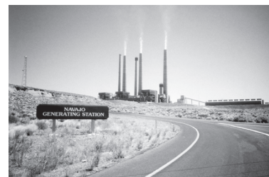
Navajo Generating Station near Page, AZ. Photo courtesy of Kim Darga.
